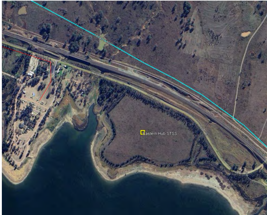
Figure 3-1 | Proposed location of the Antiene Sub Transmission Substation (STSS) 132 kV switching station
